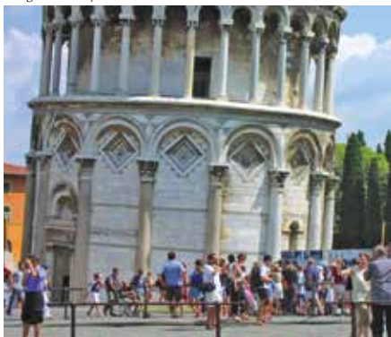
The Leaning Tower of Pisa, after John’s work, is still leaning, but more stable.
